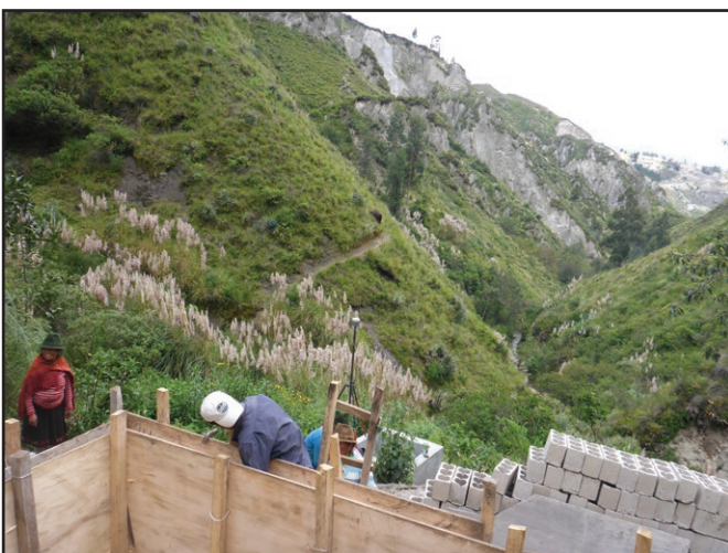
As part of the water project, Curingue residents work on building a water collection and storage structure high above the village.
