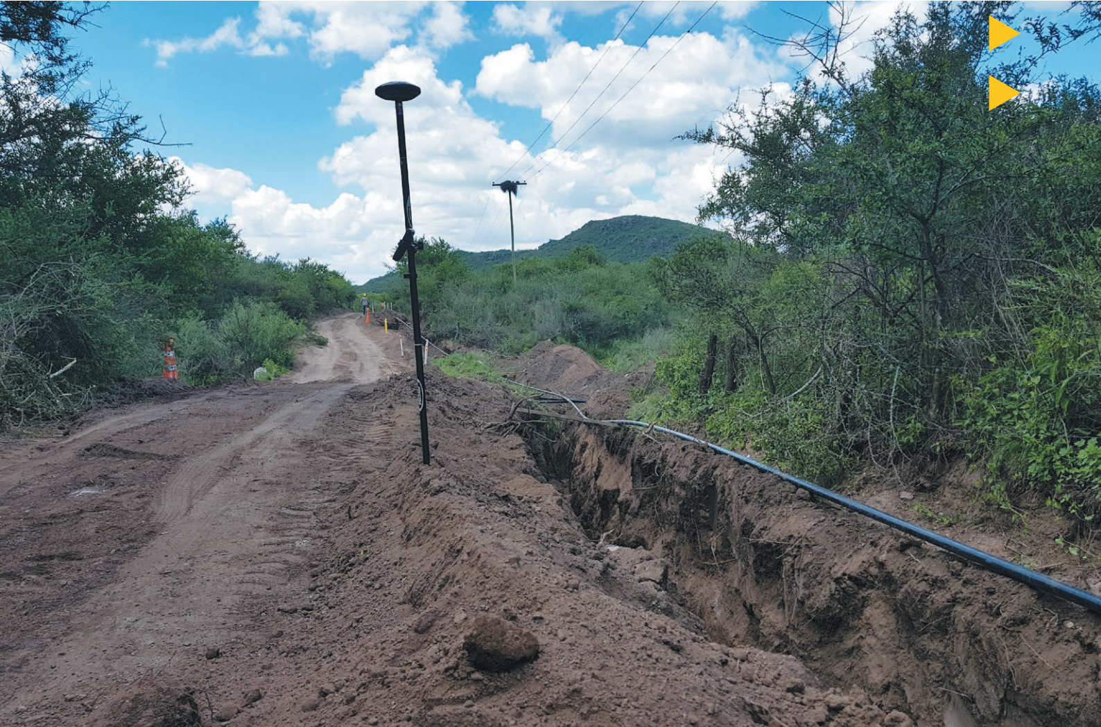
The pipeline axis is georeferenced in the construction phase to determine minimum coverage required by the pipeline.
